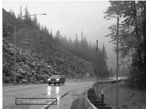
Figure 11: Poles are placed on one direction of travel to eliminate confusion
