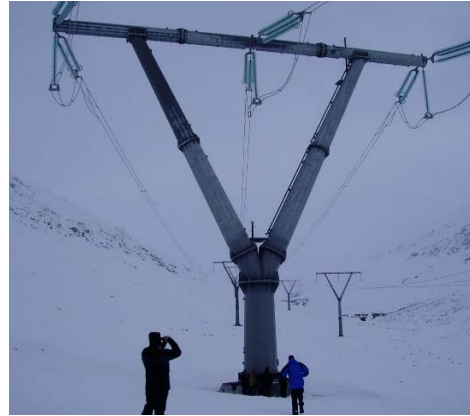
Figure 5. “Y” type Single Pole Tower
