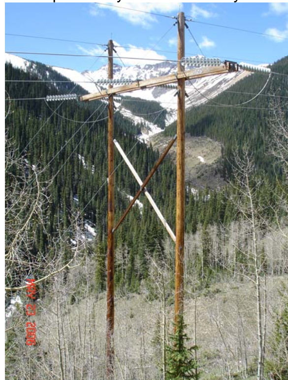
Figure 2. Structure prior to protection.
