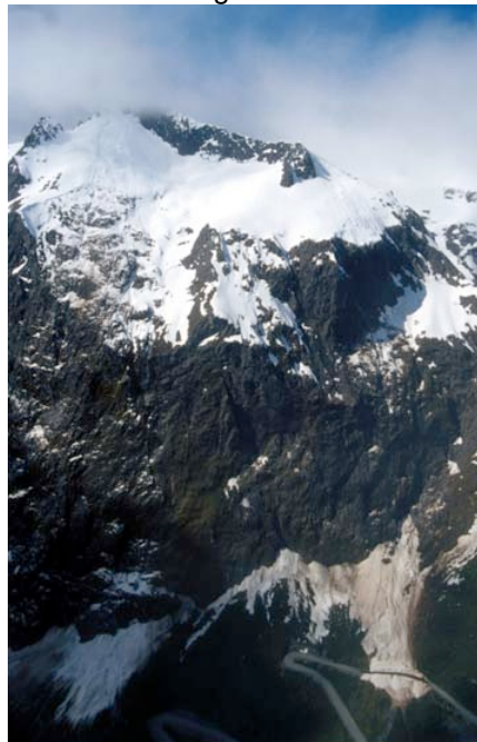
Figure 1: Aerial view of the Milford Highway. The highway traverses up the Hollyford valley, passes through the Homer tunnel into the Cleddau valley, which it follows to Milford Sound. The highway is threatened by avalanches from both sides of both valleys.
